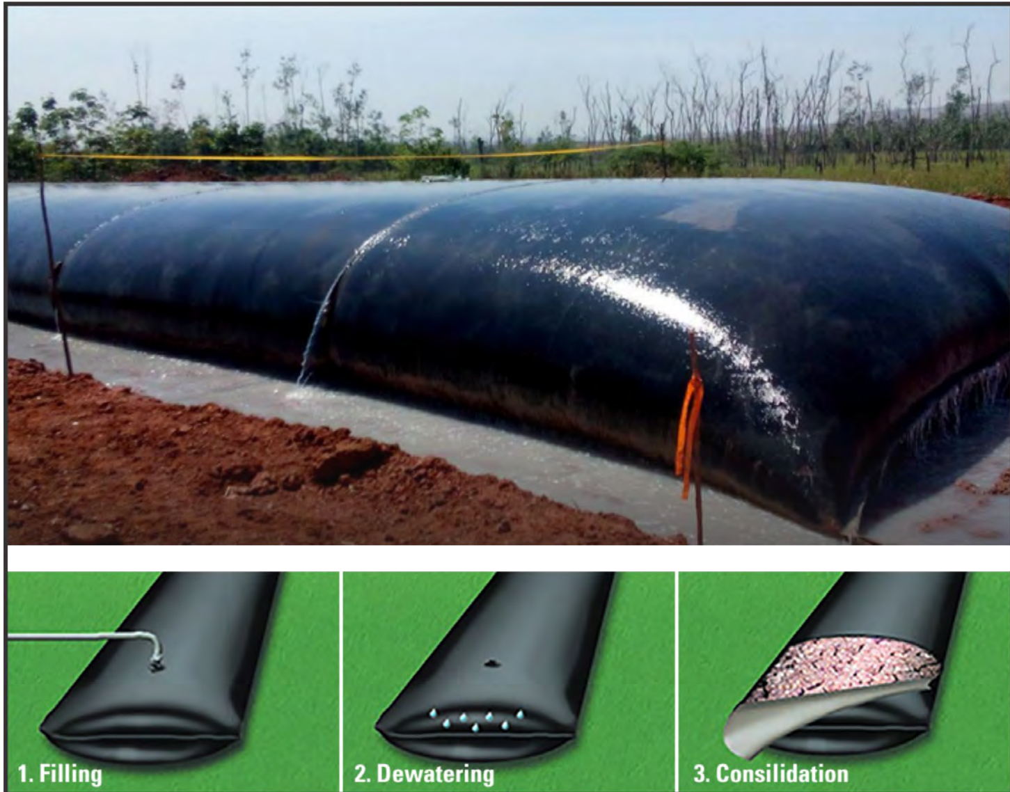
Figure 15. Example photo of a Geotube® used for dewatering sediment and how it works. Source: acigs.org and TenCate websites.
