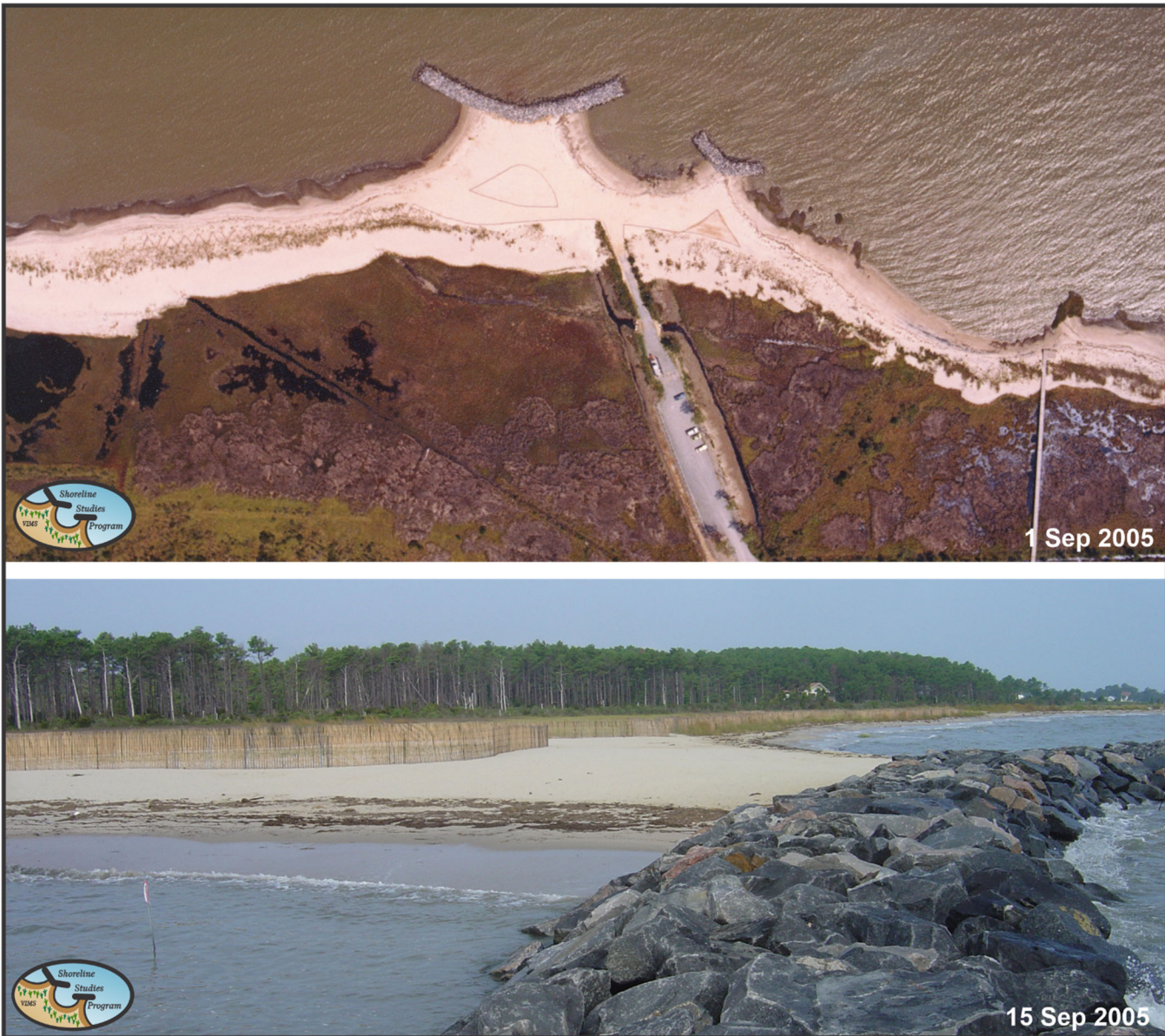
Figure 22. Aerial photo (top) and ground photo (bottom) taken at Haven Beach after breakwater and beach fill installation.
