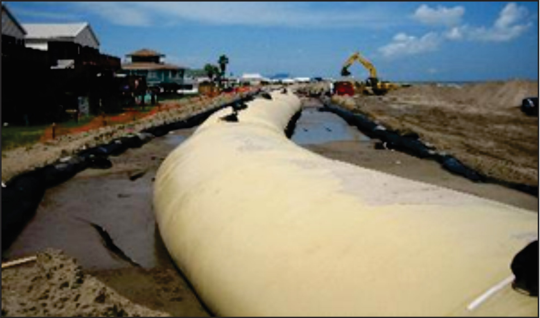
Figure 13. Example photo of a Geotube® used for sediment containment. Source: TenCate website.
