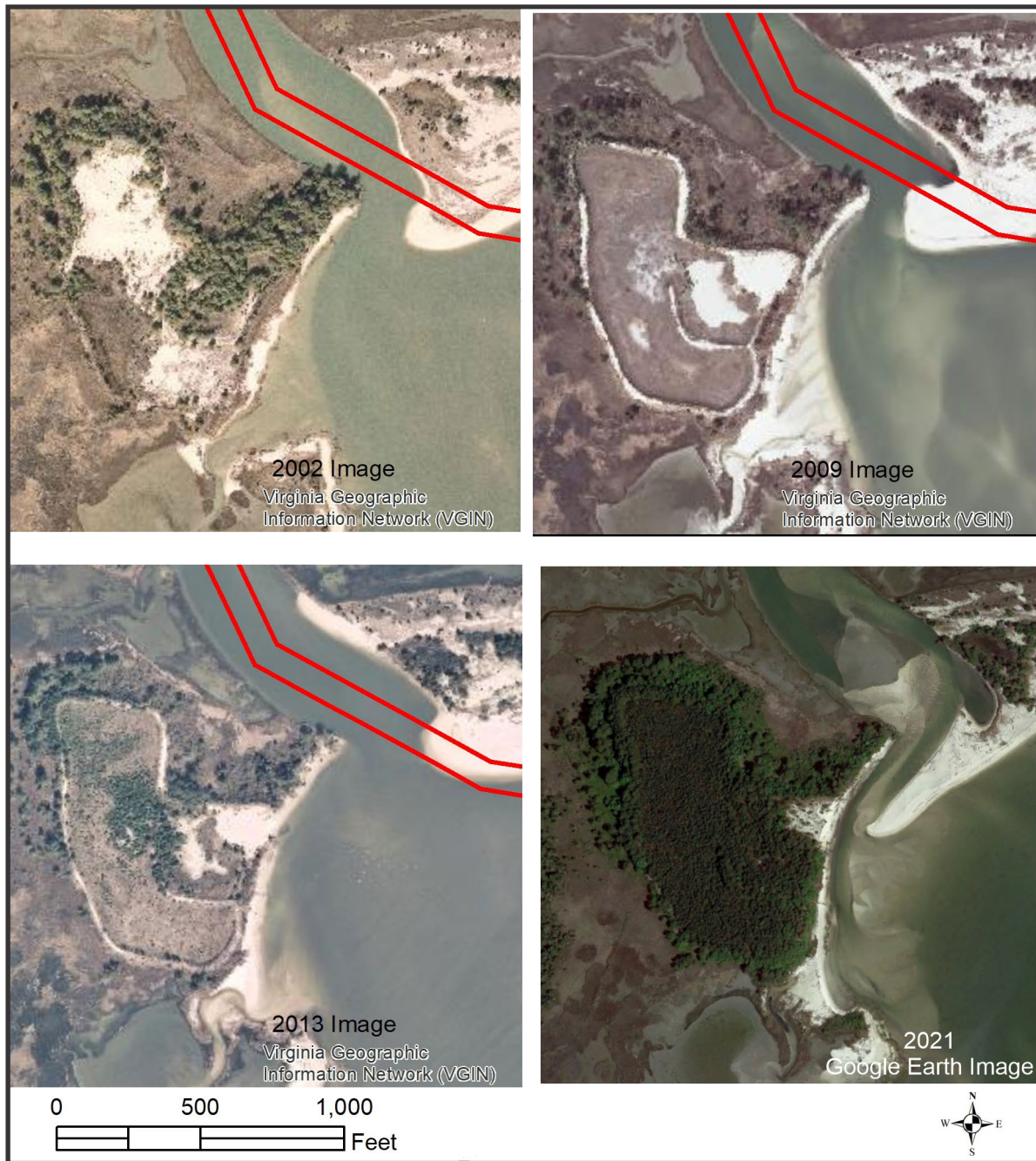
Figure 24. Aerial photos between 2002 and 2021 showing the state of the upland disposal site at Winter Harbor.
