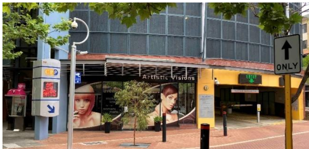
Figure 7. Parking structure. Copyright: Liang Wen.
