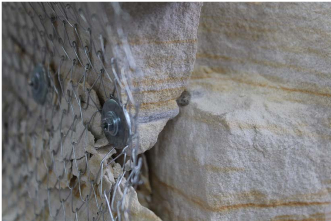
Figure 8.8 Rock bolt shear failure (after test).
