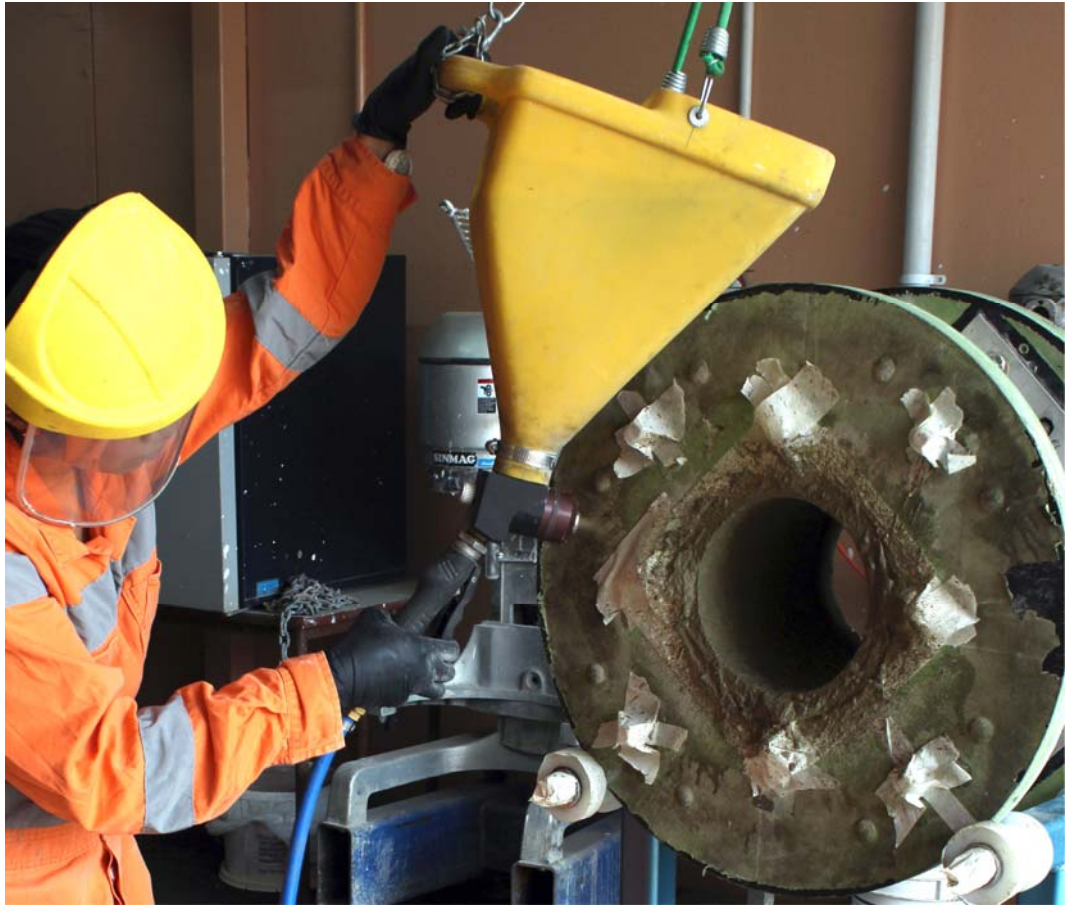
Figure 4.20 Shotcrete application by miniature spray gun.
