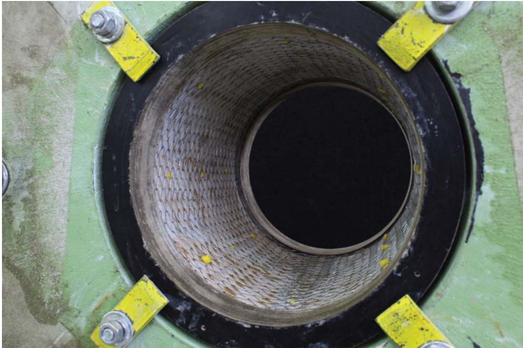
Figure 4.19 An example of a mesh installed tunnel before shotcrete application.
