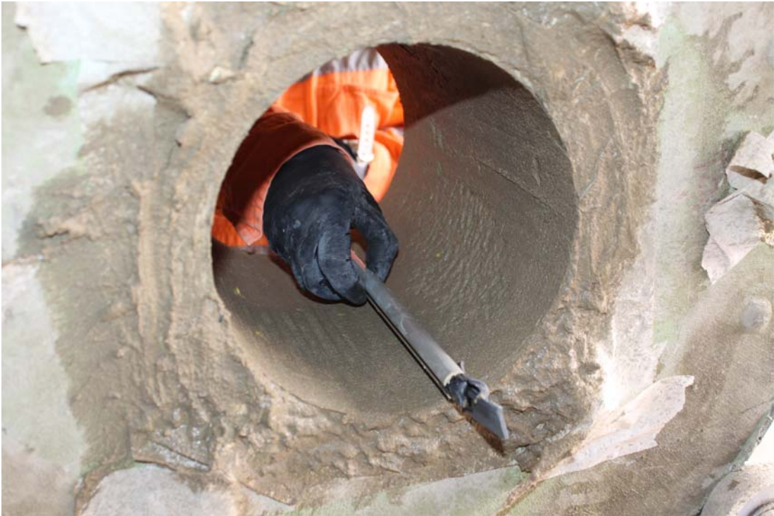
Figure 4.21 Surface smoothing process after the shotcrete spraying.
