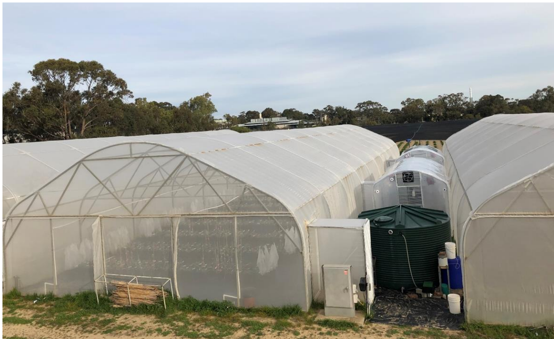
Figure 4. Birds-view of the prototype pre-breeding facility for canola heat-tolerance screening at UWA Field Station (Shenton Park, 2020). The core part of the facility are the two CERs, each with heating system, cooling system, irrigation system, and ventilation system, that are all controlled centrally. The CERs are connected to 2 screen-houses where large numbers of genotypes are grown before and after heat screening.
