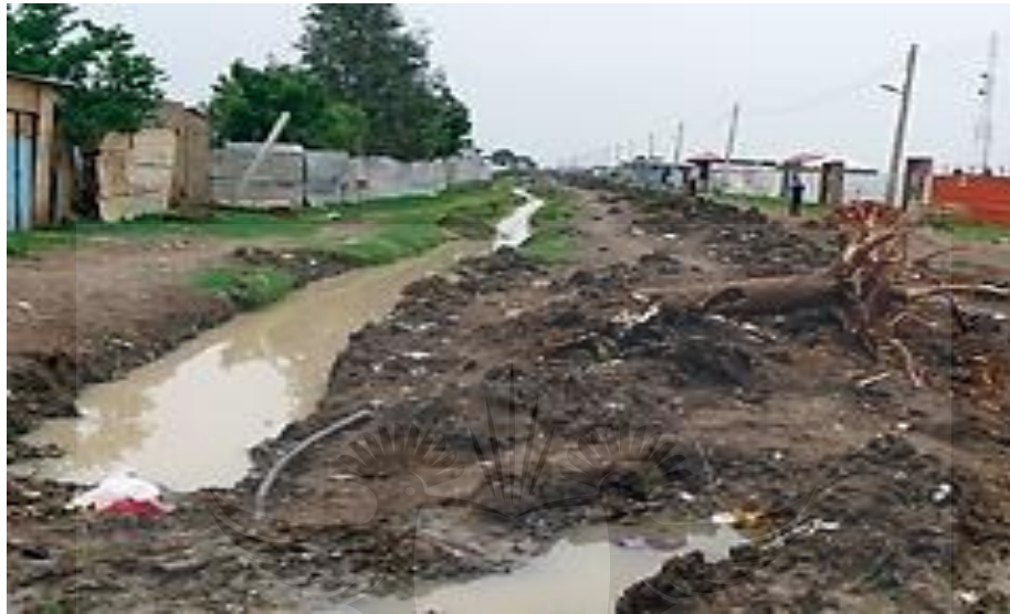
Figure 31: Impassable dirt road.
