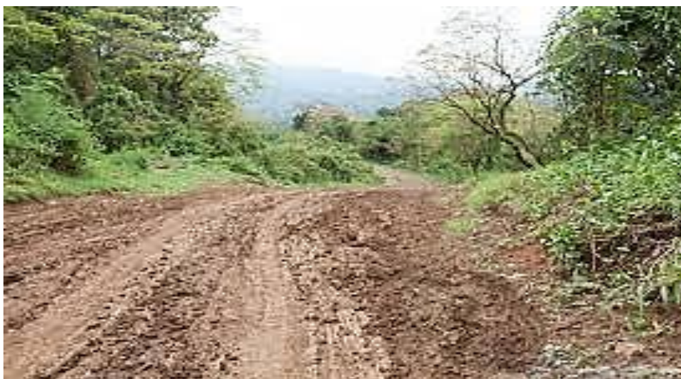
Figure 30: Slippery road surface.
