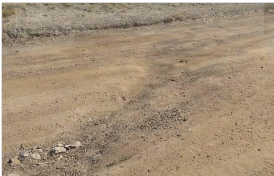
Figure 28: Erosion
