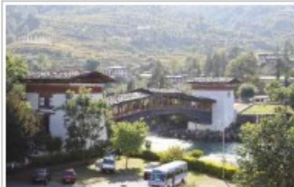
Bazem reconstructed using old anchorage buildings
