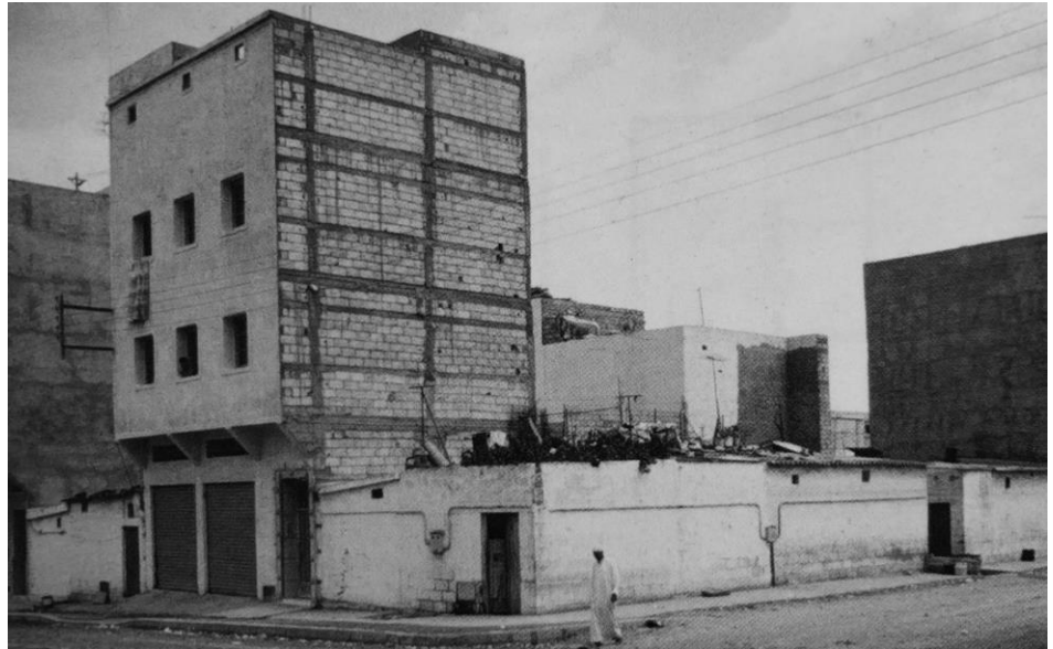
Figure 22. Growing-House. Example of block elevation in the 8x8 original patio-house. 1991. Image in: Cohen, J. & Eleb, M. 2004. Casablanca. Mythes et figures d'une aventure urbaine . Nanterre: Ed. Haza, pp. 346.
