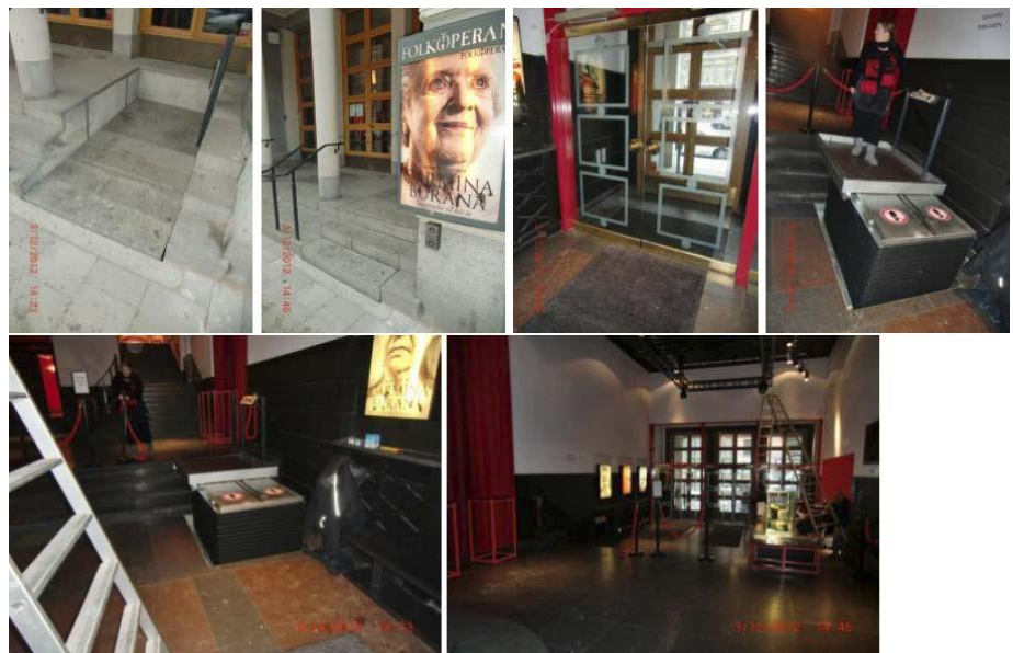
Figure 2. Overview of entrance conditions: lift tables integrated in exterior staircase, and close to inner stairs in lobby space.at the Folkoperan in Stockholm, Sweden (Photographs © author).
