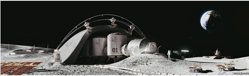
Figure 2. Artistic rendering of what a (part of a) Moon Village could look like: a habitat under a radiation shield in the centre, small rovers roaming the surface autonomously, a small telescope in the background on the left, and solar panels to supply everything with electricity. Image credit: Space is More. (Online version in colour.)
