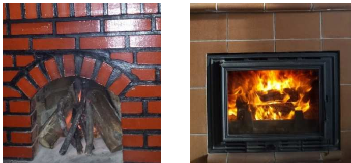
129 Figure 1. Wood combustion appliances of the present study: open fireplace (left) and 130 woodstove (right) both located in the kitchen of the households.
