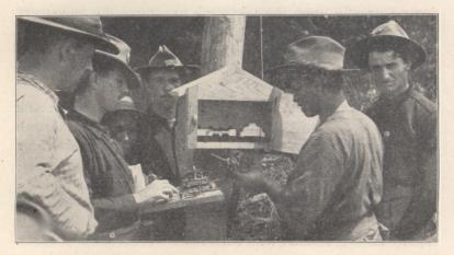
PLATE II. TESTING SUBMARINE CABLE, SHOWING CABLE BOX ARRANGEMENTS.
