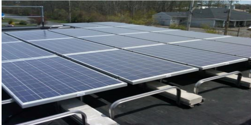
Fig 5. Flat roof mounting systems
