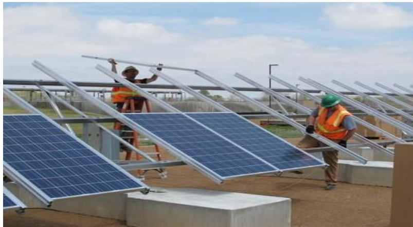
Fig 8. Panel installation
