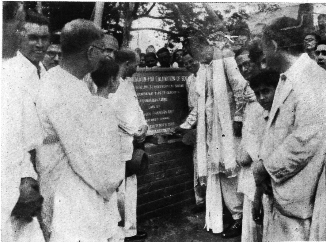
Hon'ble Dr. B. C. Roy laying the foundation stone
