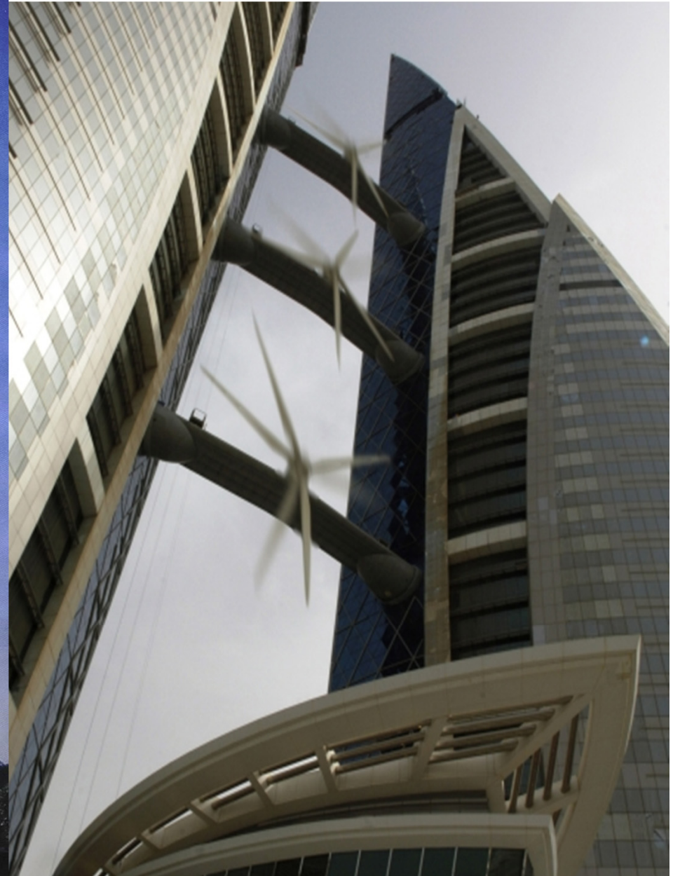
Computer generated image of the proposed world trade centre in Bahrain, one of a number of concept designs for building integrated wind turbines. www.enr.com / 2007/01/22
