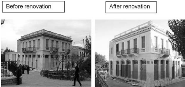
Figure 5 Restoration and façade renovation of buildings of neo-classical style and other pre-modern styles in the historical center: a case of a small neo-classical building at the corner of Eolou Street and Pelopida Street
