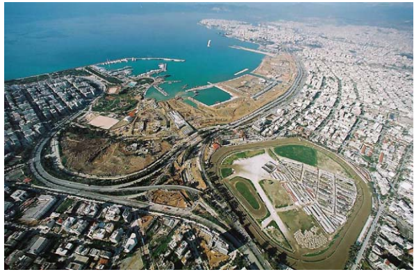
Figure 7 Waterfront redevelopment at Faliron Bay, where Olympic sports activities (beach volleyball, handball and taekwon do) will be accommodated, and the post-Olympic plans provide for the full remodeling of the area into a park hosting a wide range of sports, commercial, cultural and leisure activities
