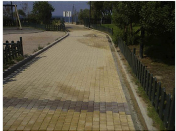
Fig. 3. A picture of the installed paving materials.
