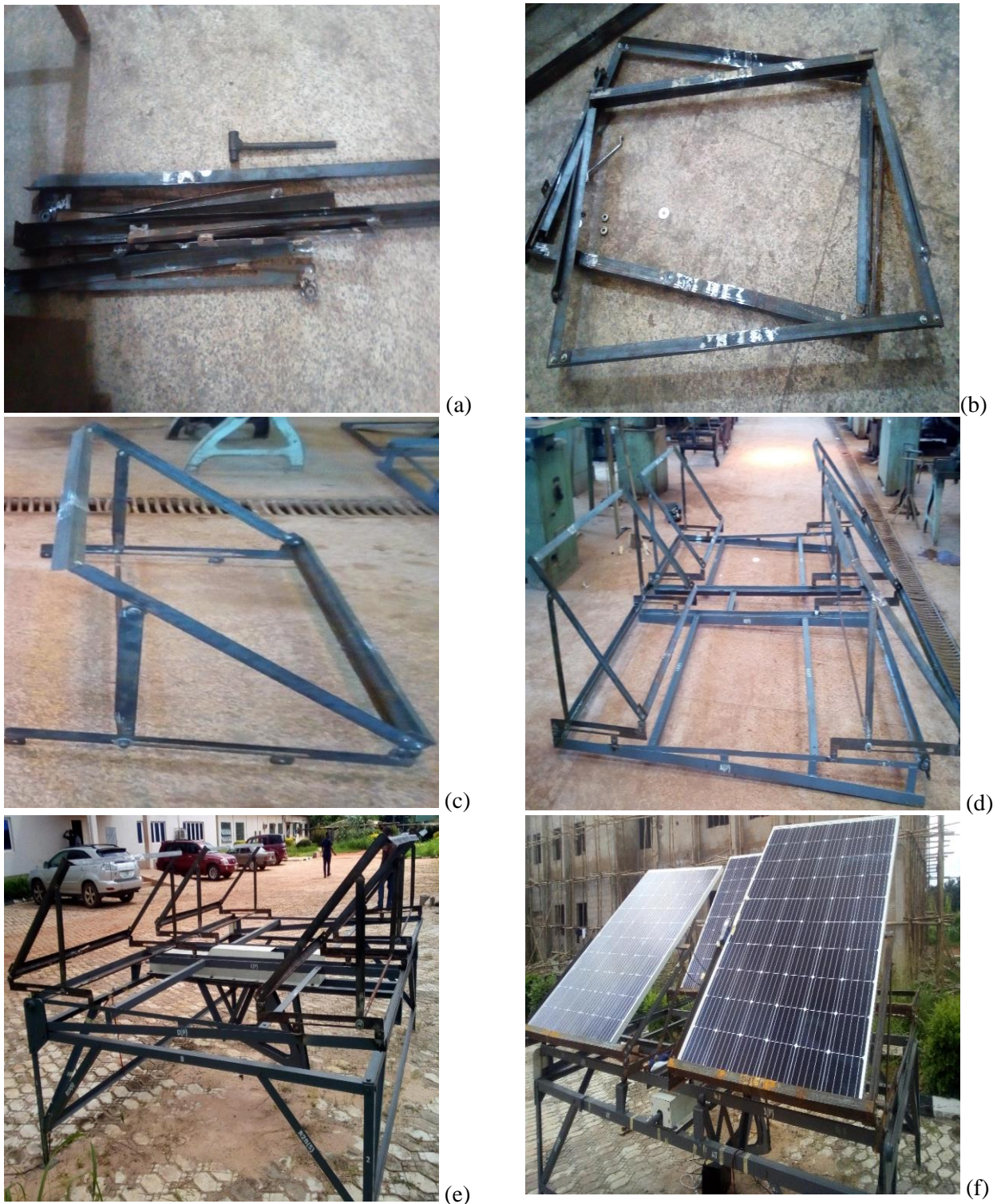
Figure 12. (a-f) The fully fabricated solar photovoltaic tilting platform prototype
