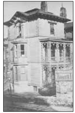
6 Alpine Street, Roxbury, site of Archer's Evening Law School, 1906-07. Archer found both a home and classroom space in this house at 6 Alpine Street, Roxbury, where he rented the ground floor. Signs for Archer's Evening Law School were displayed in the bay window.
