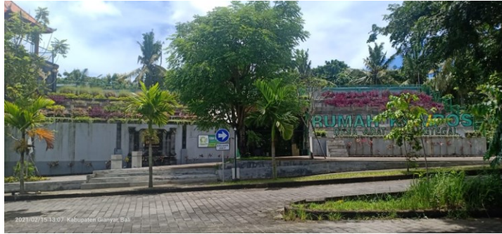
Figure 4. Monkey Forest Ubud waste processing facilities (Source: Researchers' Documentation, 2021)
