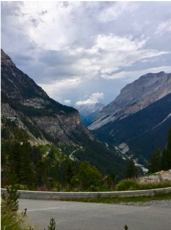
Fig. 9. The D1T road as it climbs from the Pian del Colle to the Col de l'Échelle.
