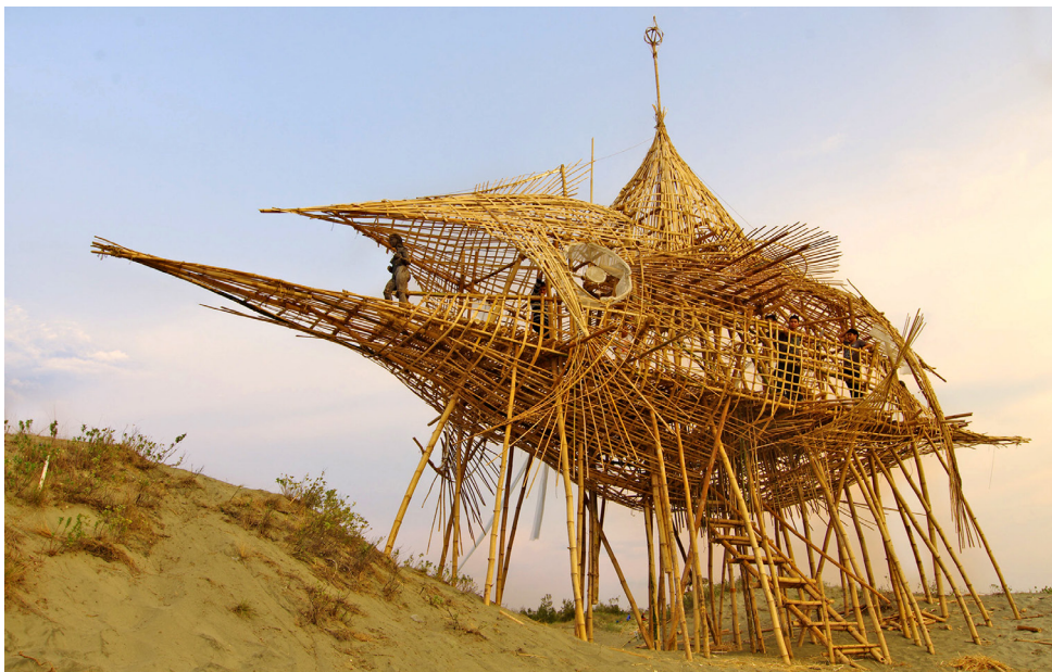
FIGURE 4: The bamboo structure is part of the Paoay sand dunes sculpture park constructed by Leeroy New in collaboration with the fisherfolk community, 2012. Image by Provincial Government of Ilocos Norte, Communications and Media Office.
