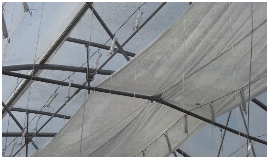
Figure 26. Plastic film placed under the roof inside the greenhouse for catching water droplets from condensation, protecting the crops (Serbia).
