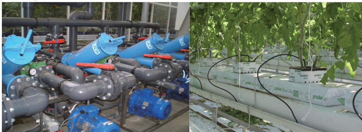
Figure 15. Drip irrigation water/nutrient solution pumps (The Netherlands), Drip irrigation system—drippers around the plants on the white gutters (the Netherlands).
