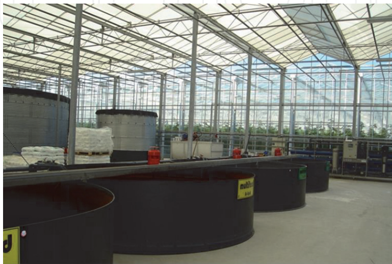
Figure 14. Tanks for water, nutrient solution, and nitric acid used for adjusting the nutrient solution pH.
