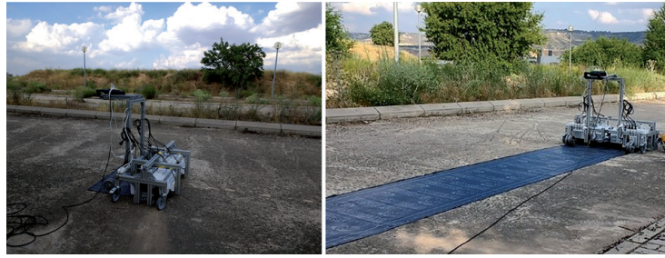
Figure 7. Outdoor installation test [17].
