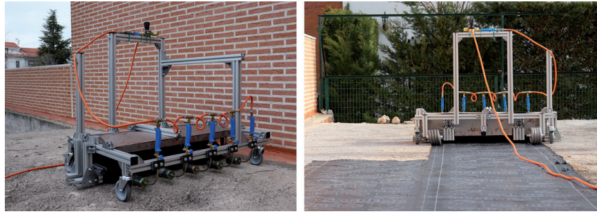
Figure 11. Prototype and results of the asphalt rolls installation.
