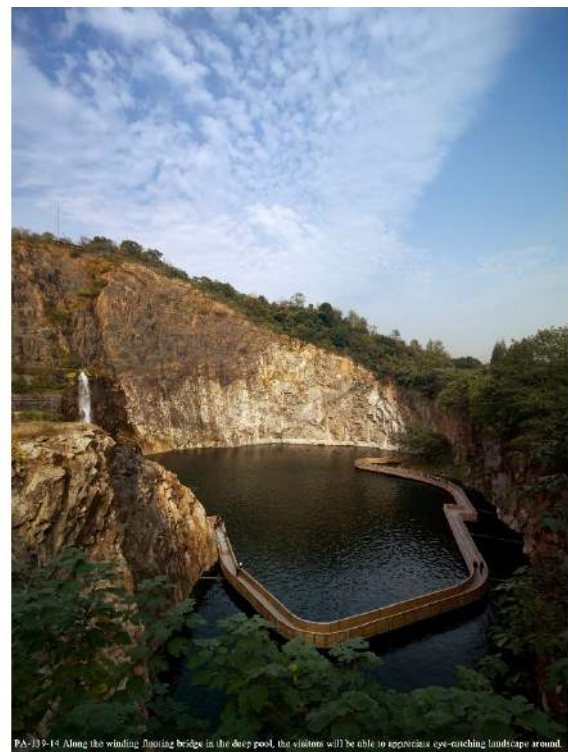
PA-139-14 Along the winding floating bridge in the deep pool, the visitors will be able to appreciate eye-catching landscape around. FIGURA 12 – FOTOGRAFIA DA RECUPERAÇÃO DO POÇO DE EXTRACÇÃO DO PROJECTO QUARRY GARDEN; FONTE: T.LY/IMHI
