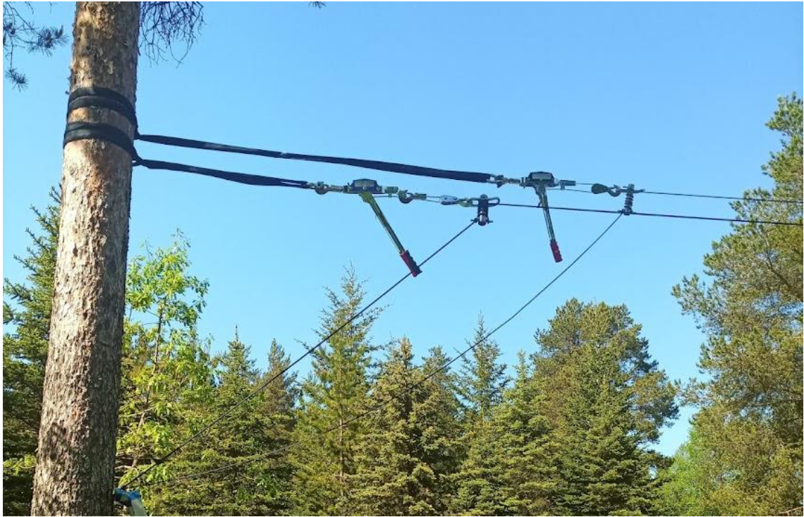
Figure 33. Installation of the cables between trees.
