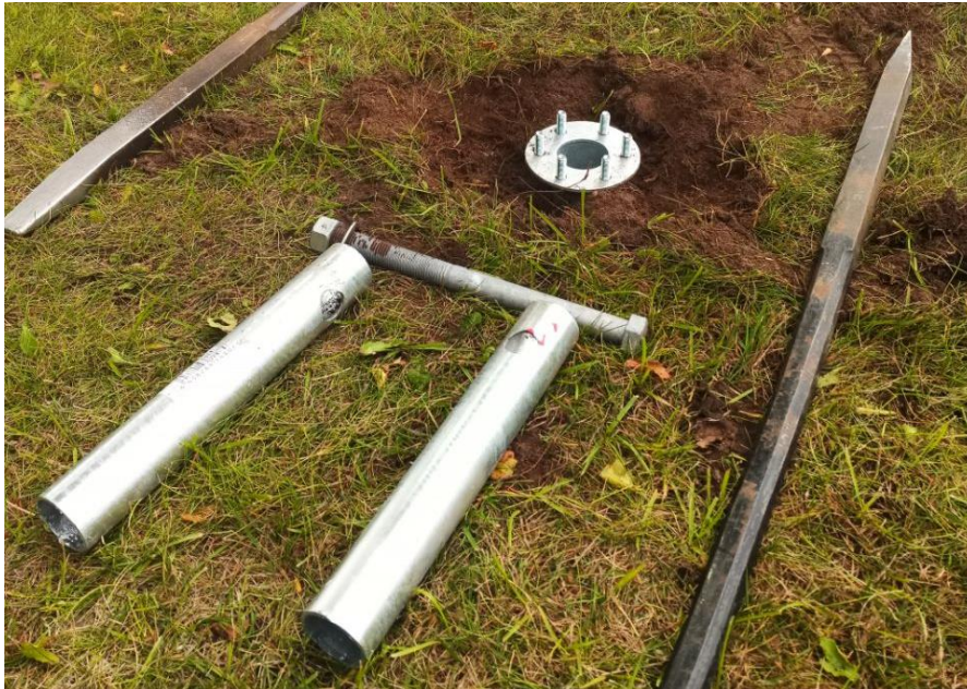
Figure 13. The screw pile and the assembly tools.
