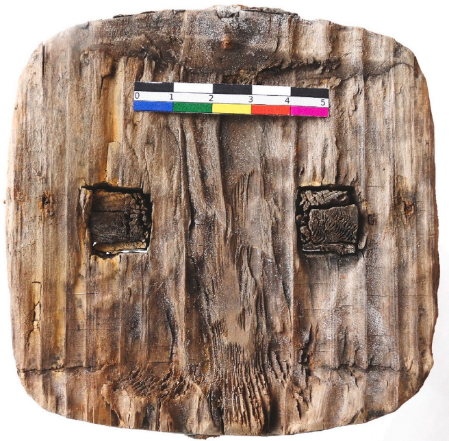
Fig. 13. Detail of the mortise and tenon joint for assembling the wooden pieces. In the upper part of the image and in the two laterals there are visible three little iron pins.
