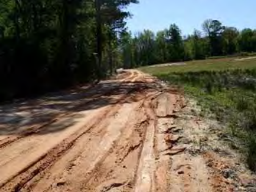
Road before work began (taken when relatively dry).
