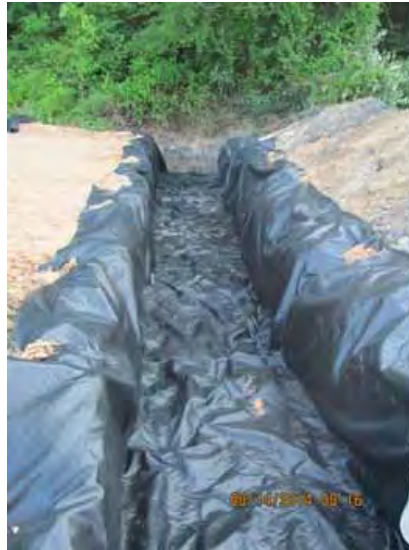
The pit is lined with geotextile fabric.
