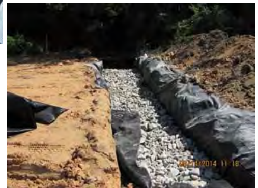
The mattress full of stone ready to be wrapped in geotextile fabric.
