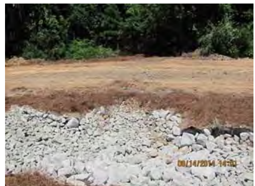
The mattress full of stone ready to be wrapped in geotextile fabric.
