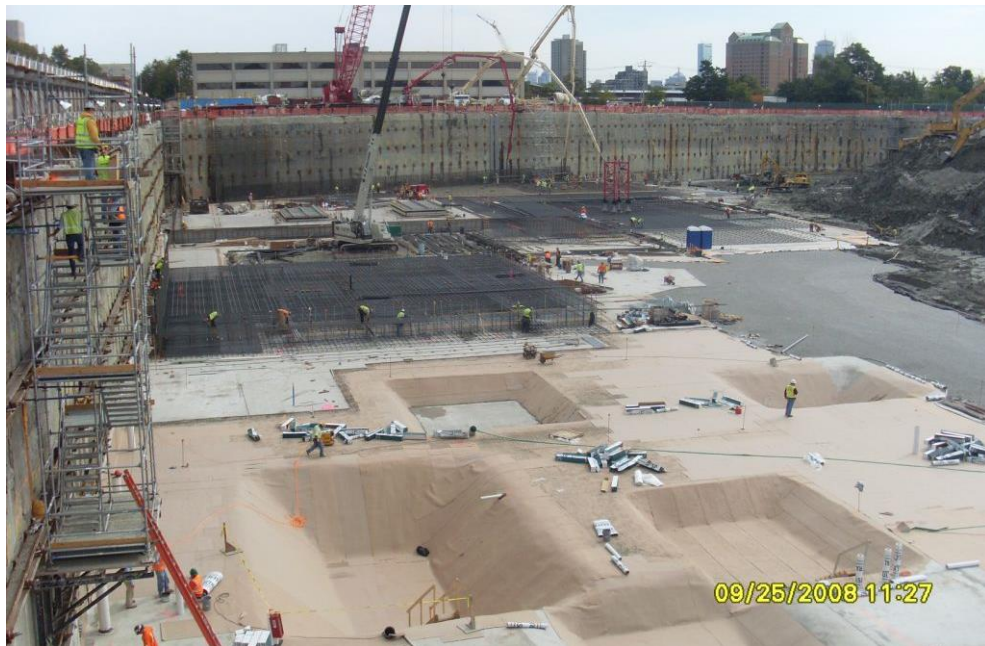
Figure 5.4 View of the site during basement excavation and construction
