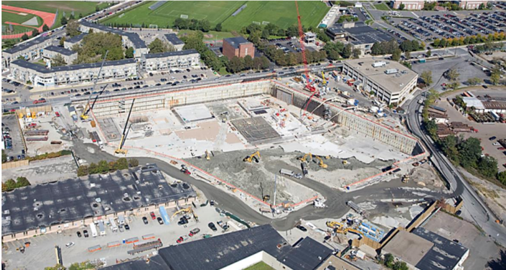
Figure 5.3 Aerial view of the site during the basement excavation works
