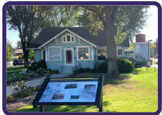
Pederson Home and Water Tower at California Lutheran University . Ventura County Historical Landmark No. 45. CC By SA-4.0.
