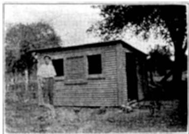
Frederick Palmtag, a Poultry Club Member, of Cherokee County, and House Built by Himself. Note Open Front on South
