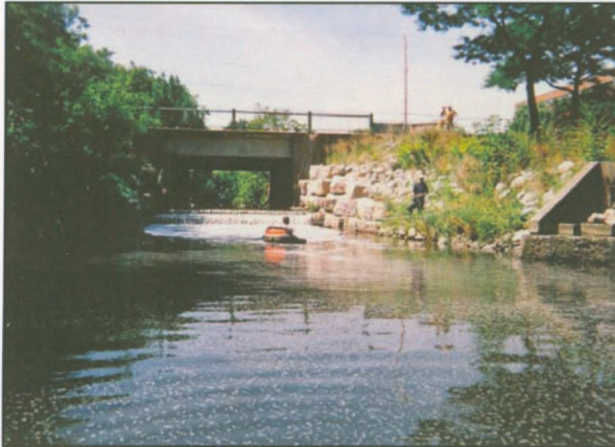
August 12, 2005: View of Crossing, Pre-Storm
