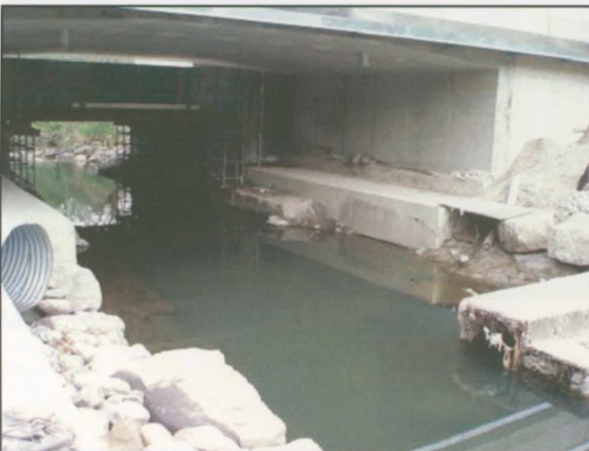
May 14, 2007: View of Crossing
