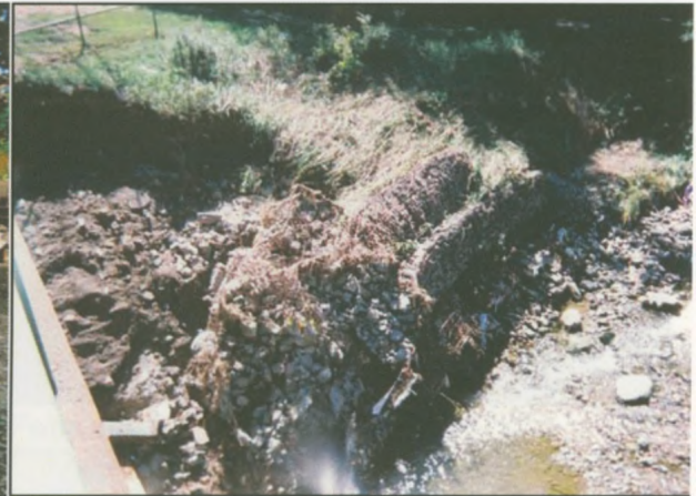
August 26, 2005: Storm Damage
