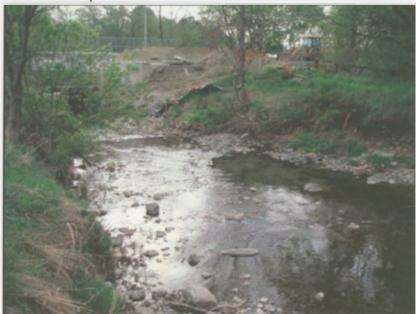
May 14, 2007: View of Crossing
