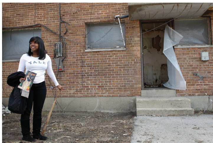
Timeica Bethel, a soon-to-be Yale University graduate, holds items she retrieved from her childhood home at the LeClaire Courts public housing complex on the southwest side of Chicago, Illinois, March 14, 2011. The complex is in the middle of demolition but she was given permission to walk through her family's unit.
