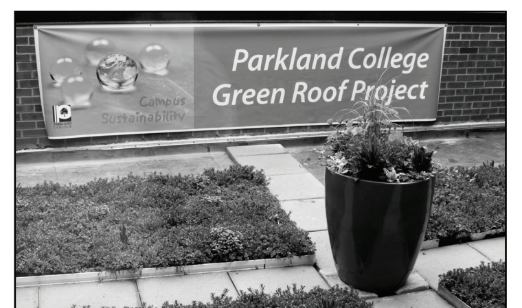
vegetation reduces hot temperatures on the roof, cutting high summer energy costs and green house emissions on the campus. Photo by Levi Norman/Prospectus News
