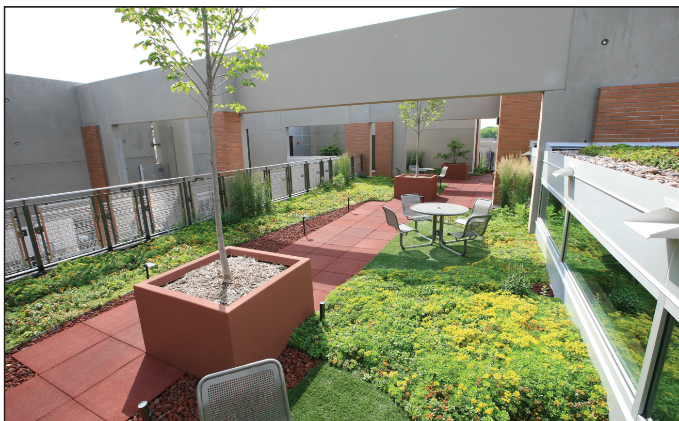
A completed LiveRoof® modular green roof system done at the Educator's Credit Union in Milwaukee, Wisconsin. Parkland will install a similar system outside of the library.
