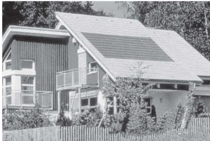
Figure 2-29 – Inclined roof with integrated PV tiles
