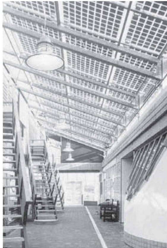
Figure 6-5 – PV cells integrated into atrium glazing (Thomas, 2003)
