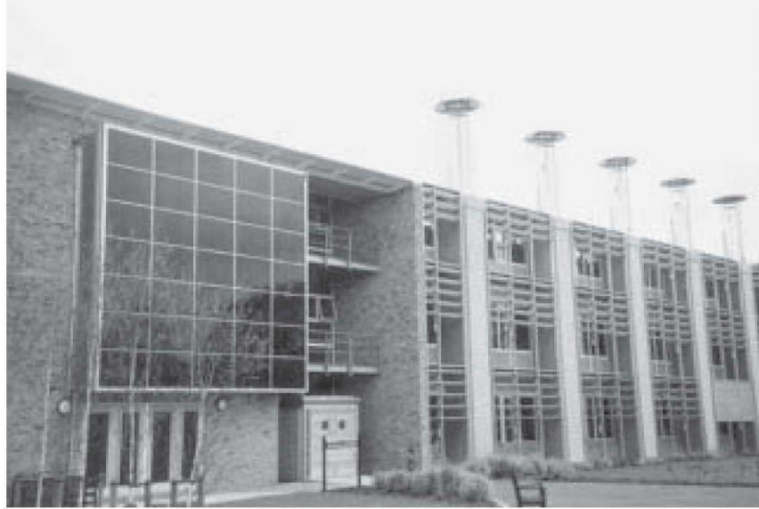
Figure 2-31 – Vertical building mounted PV array
