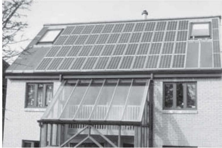
Figure 2-28 – Inclined roof with integrated PV panels
