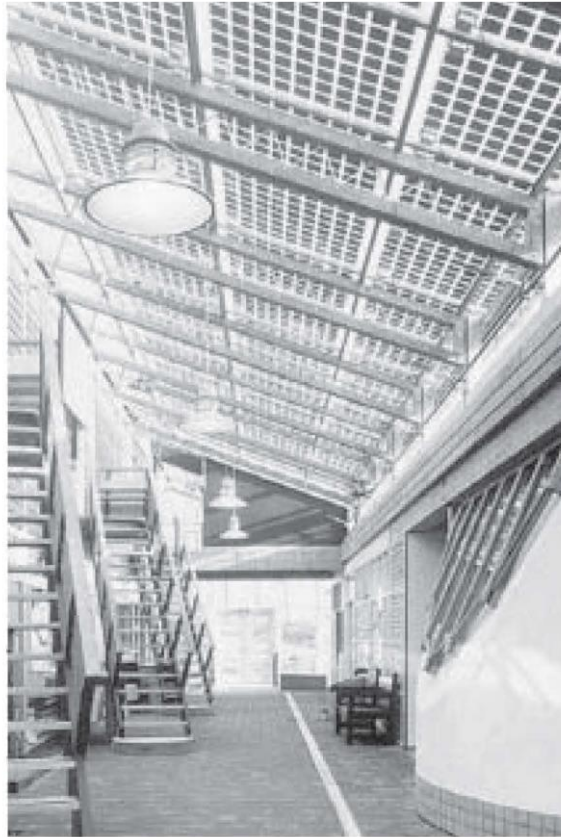
Figure 2-30 – PV cells integrated into atrium glazing (Thomas, 2003)
