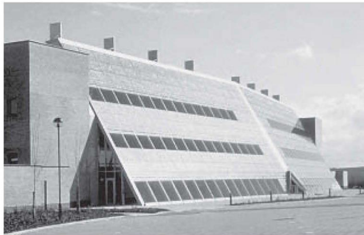
Figure 2-33 – Inclined wall with building integrated PV modules (Thomas, 2003)
