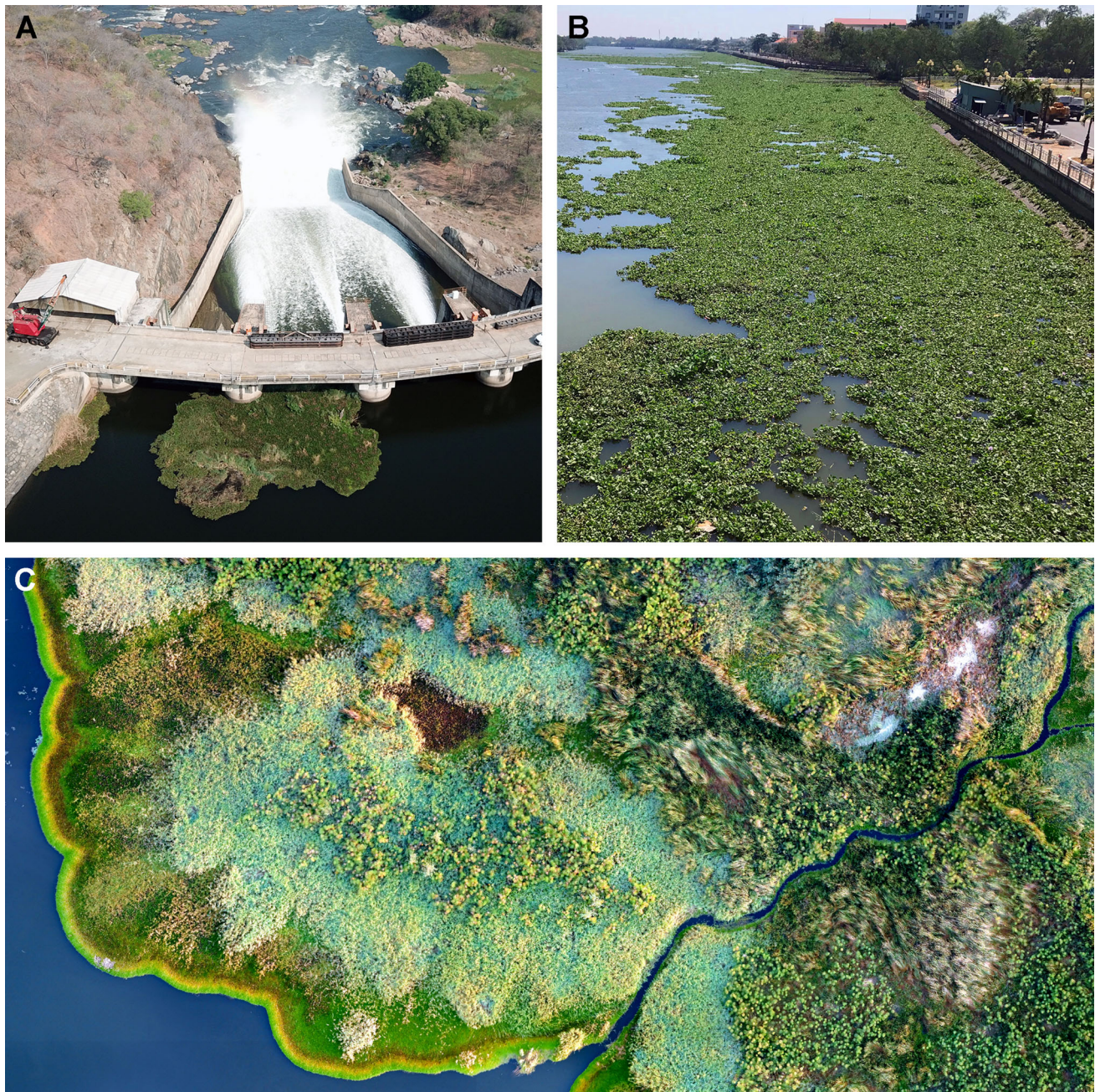
Fig. 1 A Kafue gorge dam in Zambia with floating vegetation trapped at the spillway (picture by ATEC-3D). B Carpets of floating water hyacinths on a tributary of the Vam Co Dong River in Vietnam. C Part of the Kafue flats wetland in Zambia. The bright green fringe along the shore is composed of two exotic floating plant species, water hyacinth and Amazon frogbit (picture by ATEC-3D)
