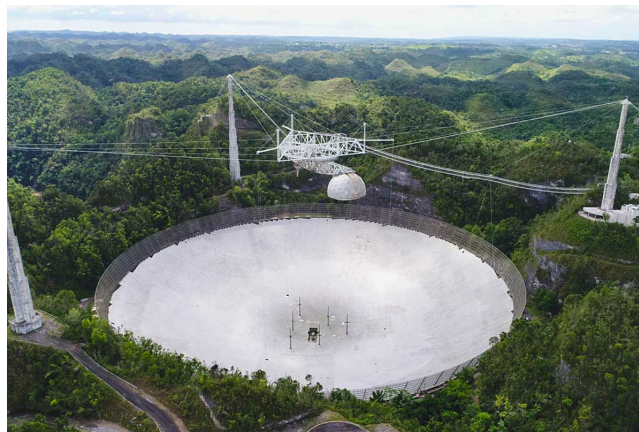
Figure 1.2: Arecibo Telescope, the second largest radio telescope. In this scale, almost all steerability of the telescope is lost. From ucf.edu
