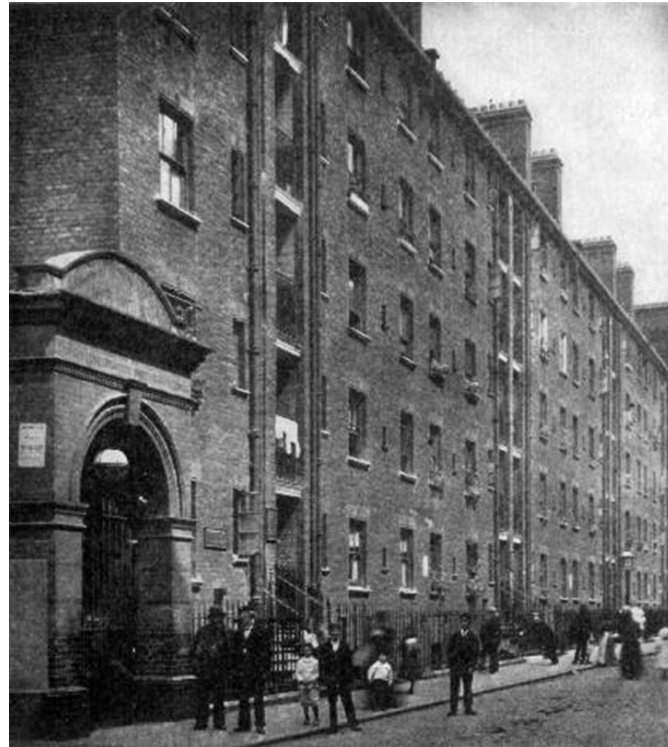
Figure 5.6: Thrawl Street, showing a typical ‘monotonous’ facade
