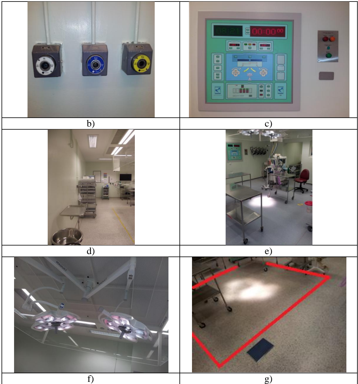
Figure 5.3 The various characteristics of the operating theatre: a) gas outlets and vacuum pressure, b) master control panel, c) Space surrounding operating area and diverse medical equipment, d) distribution of equipment around operating area, f) lightning, g) operating area.
