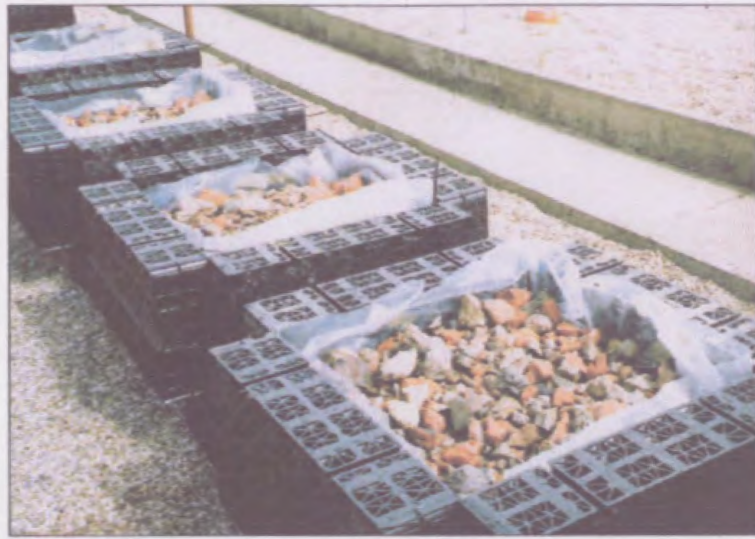
Figure 11b Addition of the recycled aggregate sub-base material to the rig
