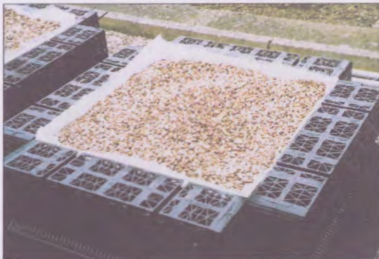
Figure 13 The gravel layer
