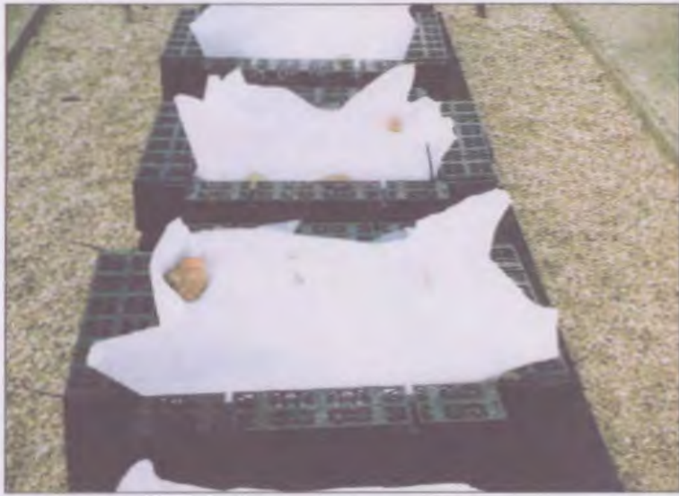
Figure 12 Separating the gravel layer from the sub-base
