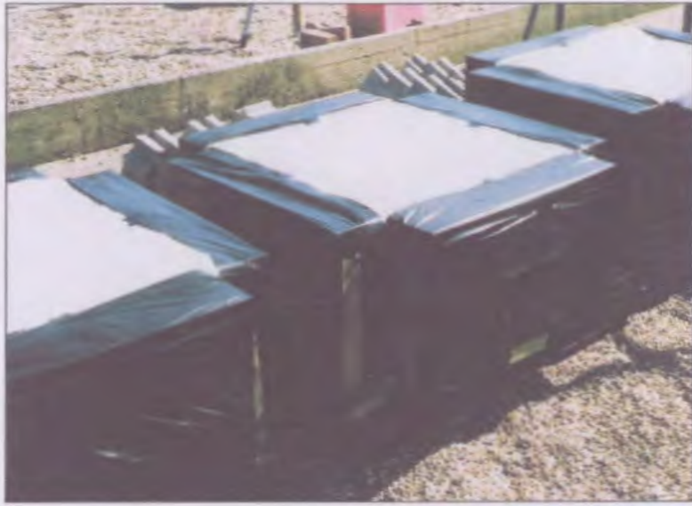
Figure 14 An additional layer of geotextile
