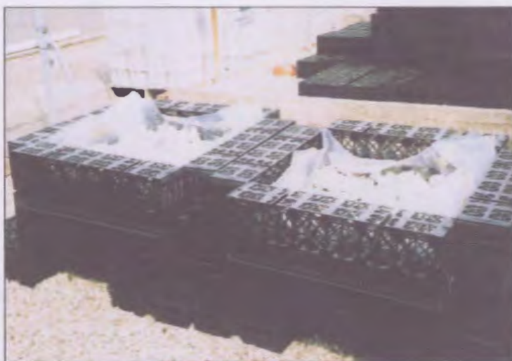
Figure 11a Addition of the granite sub-base material to the rig
