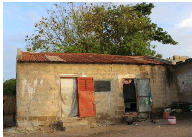
Figure 123. Brick, cement, and corrugated iron sheet construction in Ndiémane © Carla Sarrouy Kay 2019
