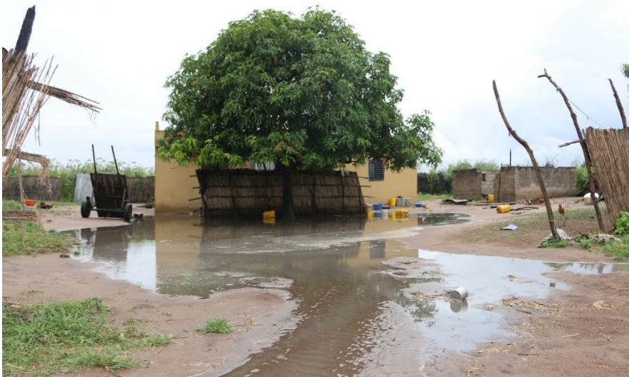
Figure 88. Concession flooded after a strong cloudburst at the end of the rainy season, October 2019 © Carla Sarrouy Kay 2019
