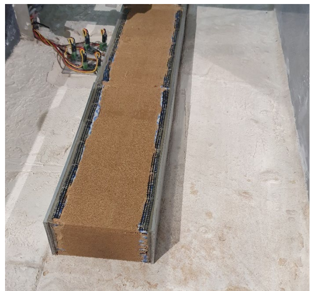
Figure 1. A section of 1/50 th scale (50mm high) geosynthetic reinforced soil retaining wall (GRS-RW) embankment under construction in the centrifuge rail simulator, on a soft clay subsoil.
