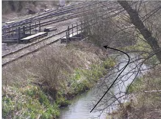
Figure 2.17 Watercourse passing under a track through a culvert (Network Rail, 2010)
