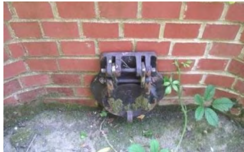
Figure 2.16 Flap valve (Network Rail, 2010)
