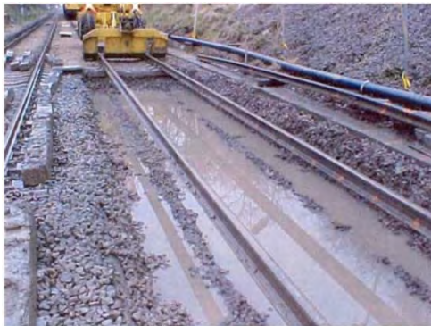
Figure 2.18 Wet beds (Network Rail, 2010)
