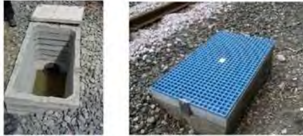
Figure 2.10 Typical catchpits (Network Rail, 2010)
