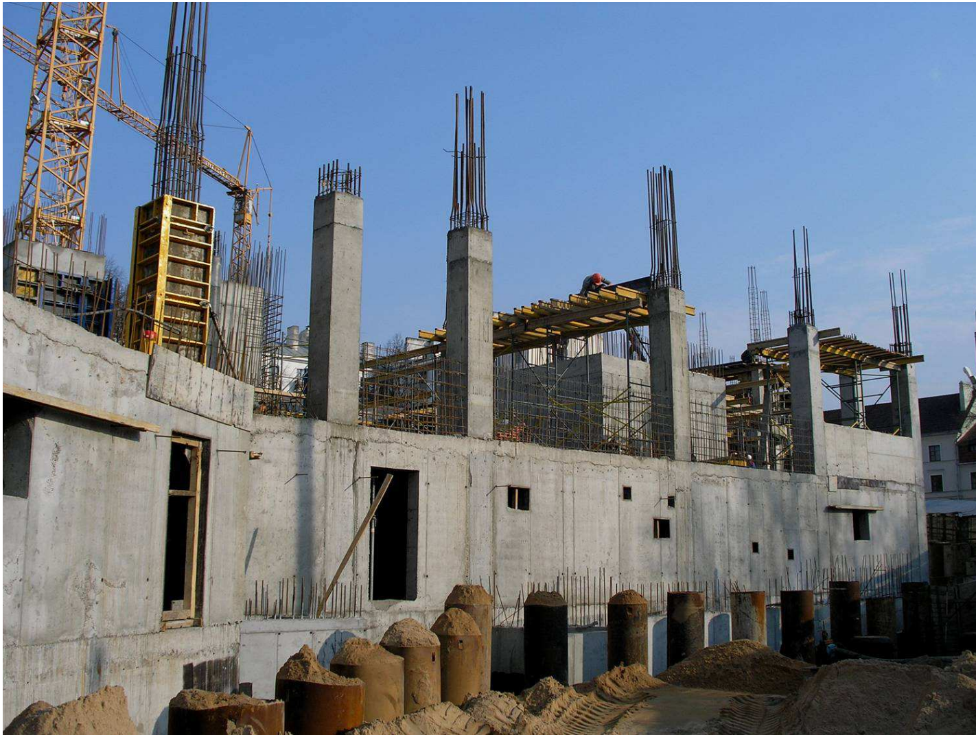
Pic. 25. Construction of the building from a monolithic reinforced concrete
