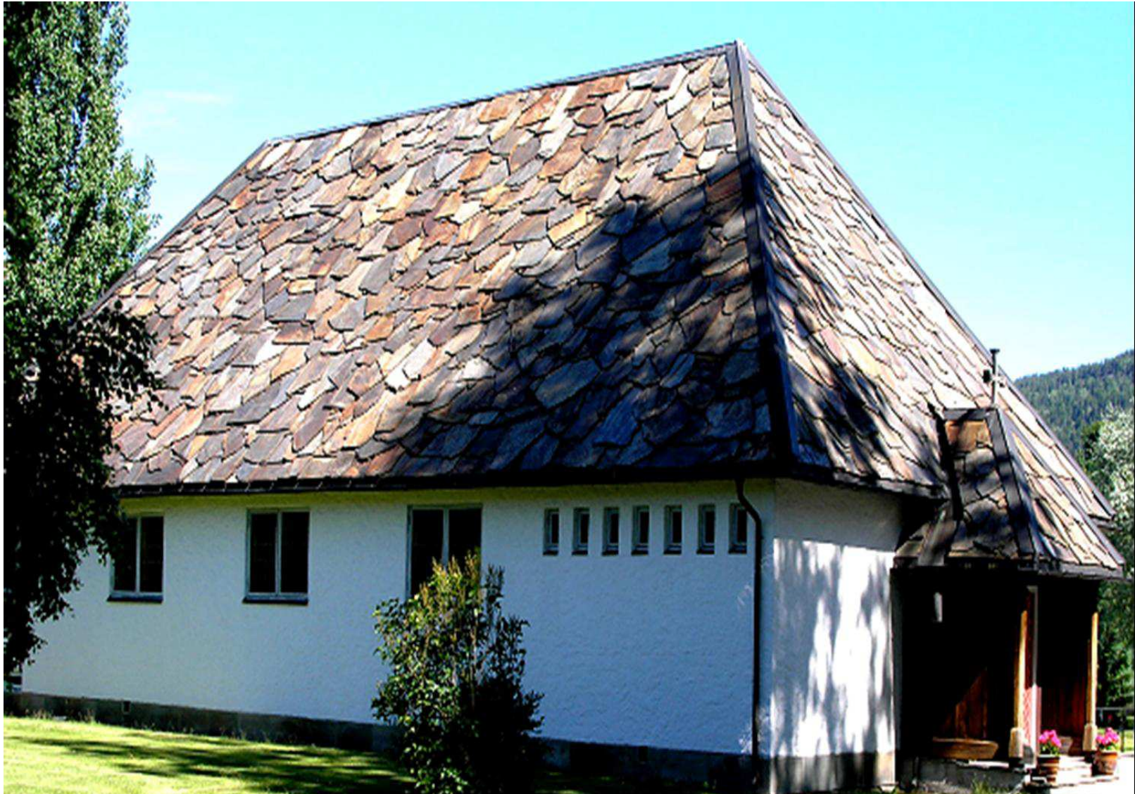
Pic. 12. The roofing materials from clay shales
