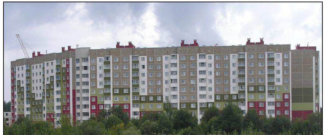
Pic. 26. Construction of buildings from wall panels
