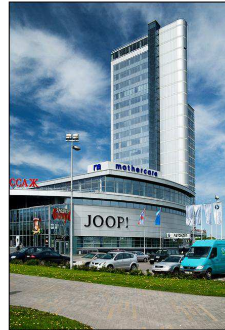
Pic. 18. Construction and application of glass slabs
