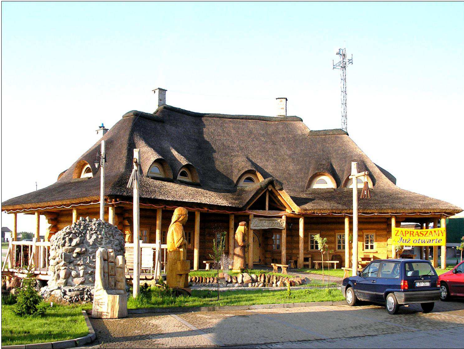
Pic. 2. The use of reed as roof material
