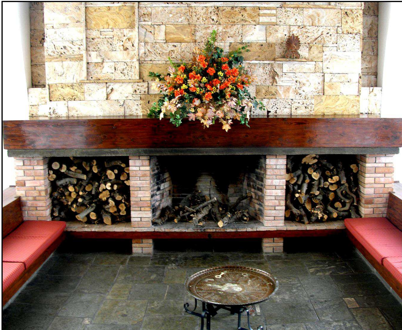
Pic. 11. Facing slabs for floors and interior walls from natural rock
