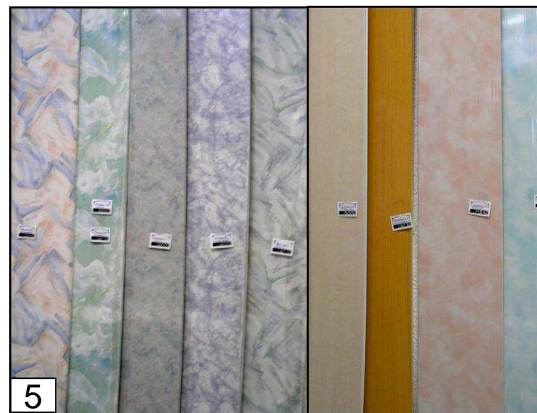
Pic. 4. Organic materials for finishing interior walls and ceilings: 1,2 – wallpaper; 3 – acoustic board from polymer materials; 4 – decorative veneer; 5 – panels from polymer materials.
