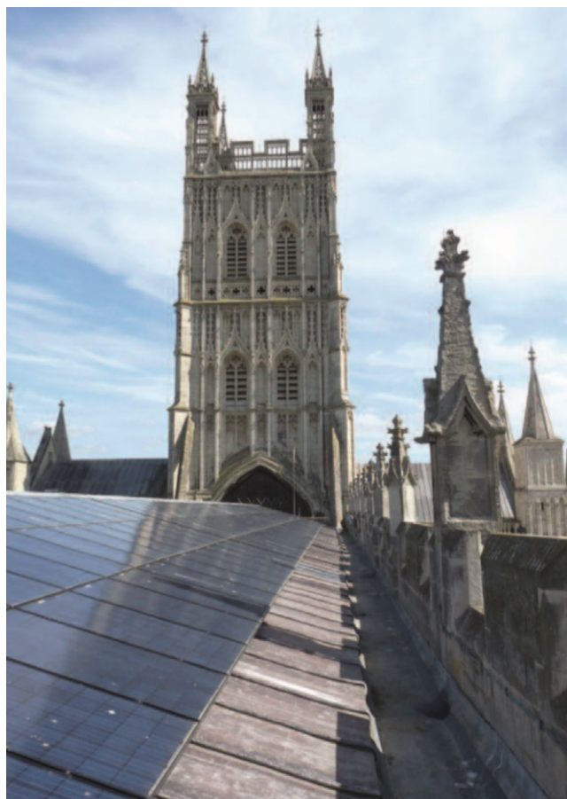
FIGURE 1 A view of Gloucester Cathedral roof upon completion. Image provided by Mypower Solar 15
