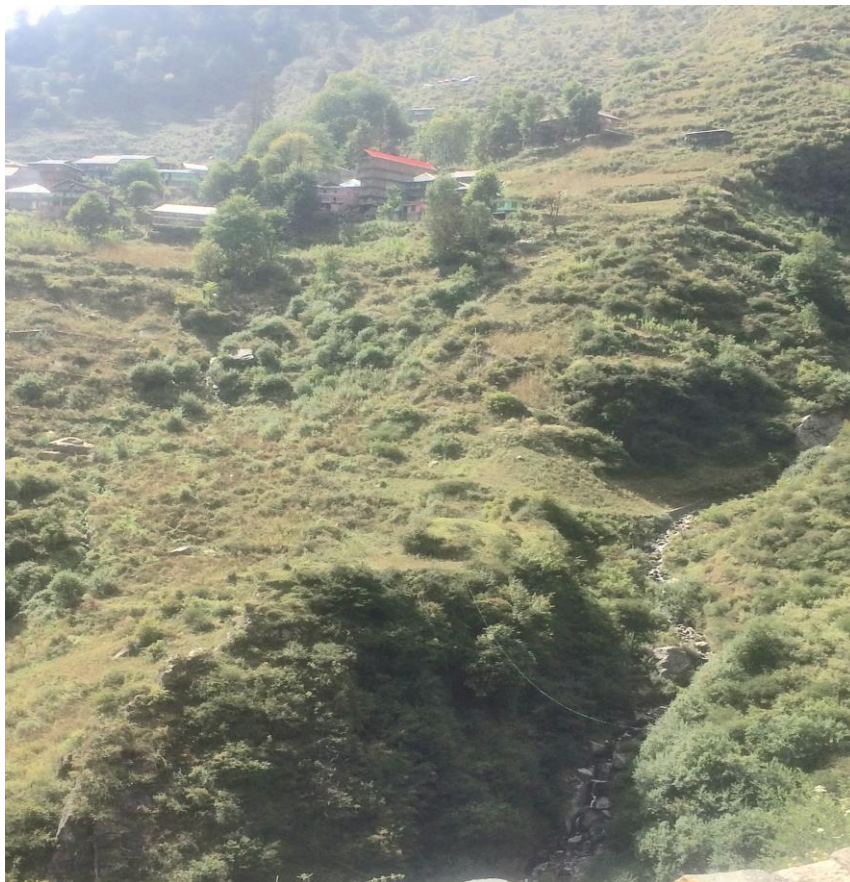
Figure 7.1 shows houses in the Malana village scattered along the mountain
