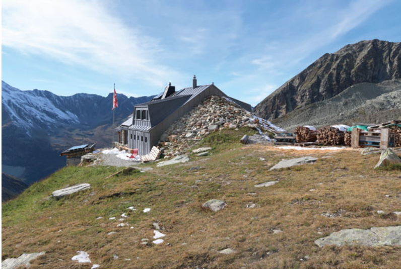
Figure 3. Photograph of a snow avalanche defence built against the Cabane Arpitettaz near Zinal, Switzerland. The geometry of boulders built up against the structure resembles a maximal pile (§ 7), which is a stable shape that effectively diverts incoming snow away from the building.
